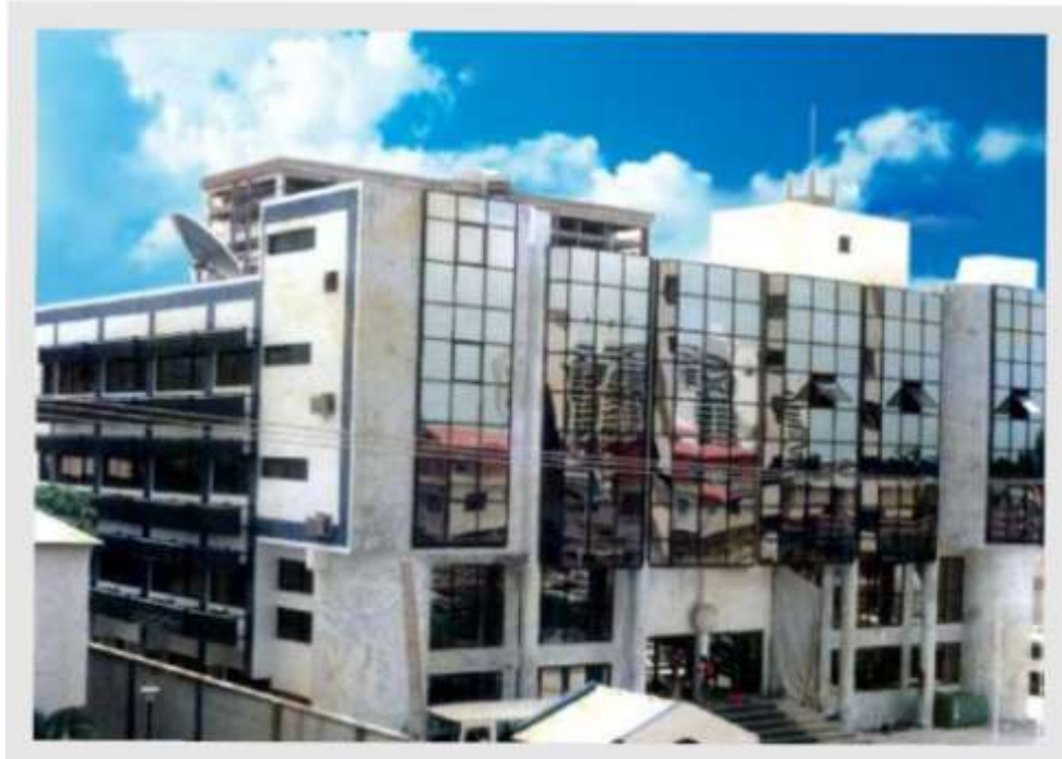
(STRUCTURAL ENGINEERS & SUPERVISORS) ALL STATES TRUST BANK, OYIN JOLAYEMI STREET, V.I, LAGOS STATE
